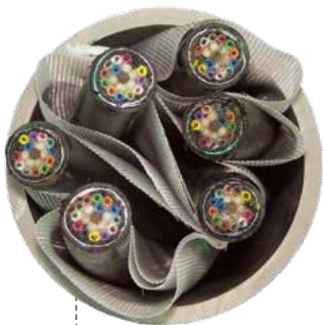
4" 3-Cell packs with 6 1" OD cables in 4" conduit
