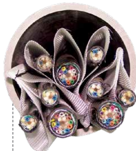
3" 3-Cell packs, 9 cables in 4" conduit
