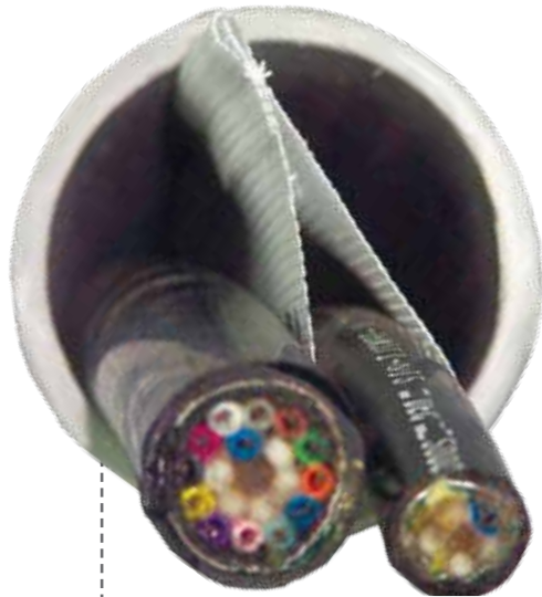
2" 1-Cell MaxCell overriding incumbent cable in 2" conduit
