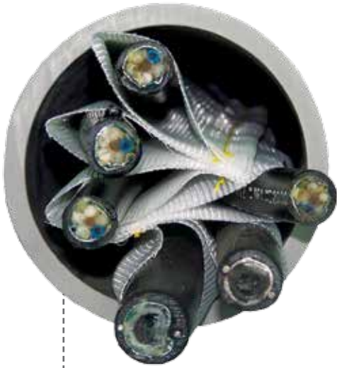
2" 3-Cell packs, 6 cables in 3" conduit
