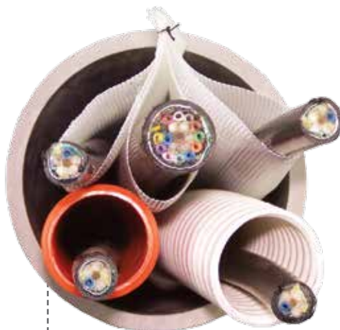
3" 3-Cell pack overriding existing cable plant in 4" conduit
