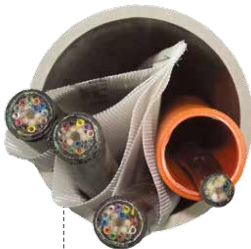
4" 3-Cell packs overriding existing cable plant
